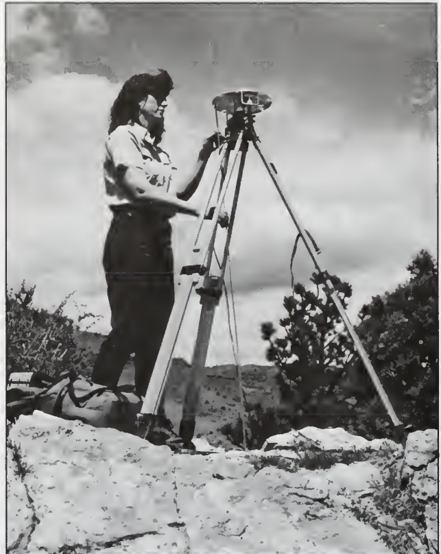
Figure 21. A land surveyor measures the height of a Global Positioning System (GPS) antenna. The antenna is mounted on a tripod, which has been precisely set up over a survey point with a known location. Once the measurement is made, the receiver is turned on and data collection begins.
